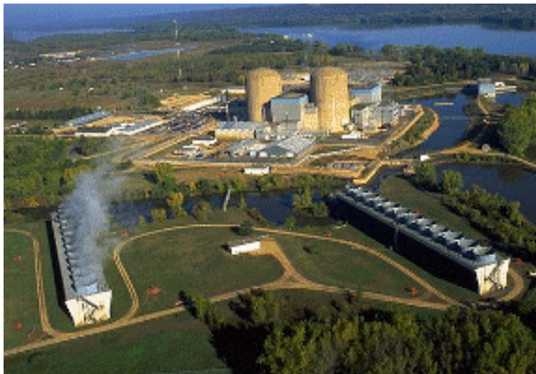
Figure 7: Typical Mechanical Draft Cooling Towers
